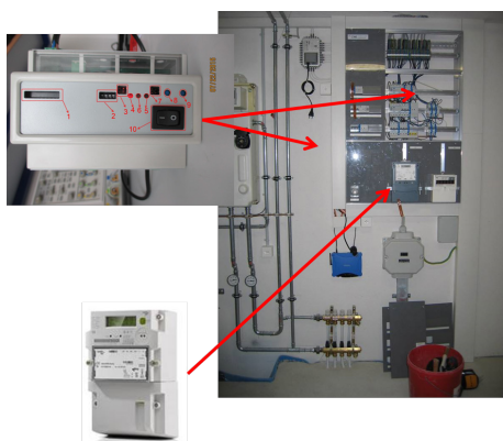
Figure 3: Installation of Prosumer Household Measurement and Control Equipment (above: GridSense box, below: L+G 350 SmartMeter)
